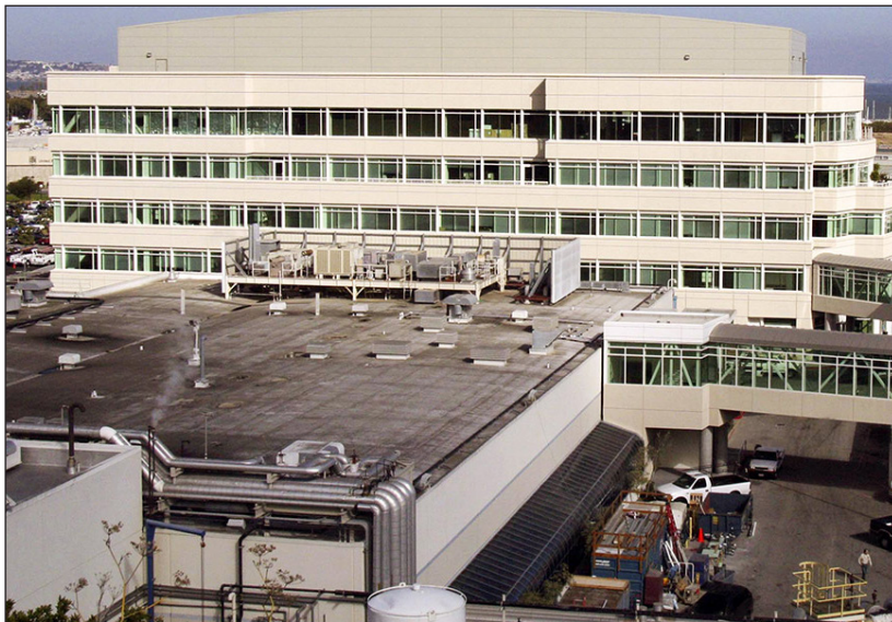
Lower Campus R&D and Manufacturing Space
